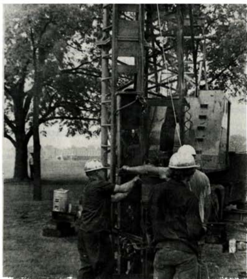
FIGURE 2 - INSTALLATION OF FORCE TRANSDUCER
