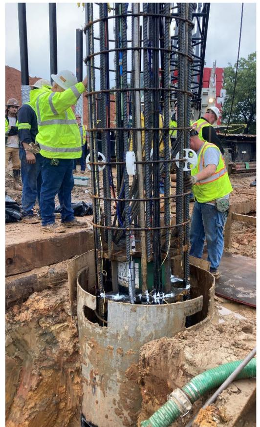
The bi-directional static load test applied a maximum unidirectional jack assembly load of 2,152 kips and a maximum test load of 4,304 kips. Measured strains were converted to internal forces using the [Incremental Rigidity Method](#). These results, combined with the interpreted cross-sectional areas determined from Thermal Integrity Profiling, were used to assess the unit shaft resistance along the length of the tested shaft.
