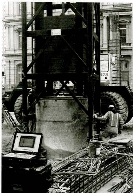
Figure 1. 40 ton drop hammer on 78" diameter shaft with PDA in foreground
