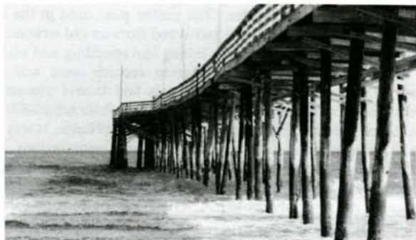
Figure 1: General View of Pier and Piles
