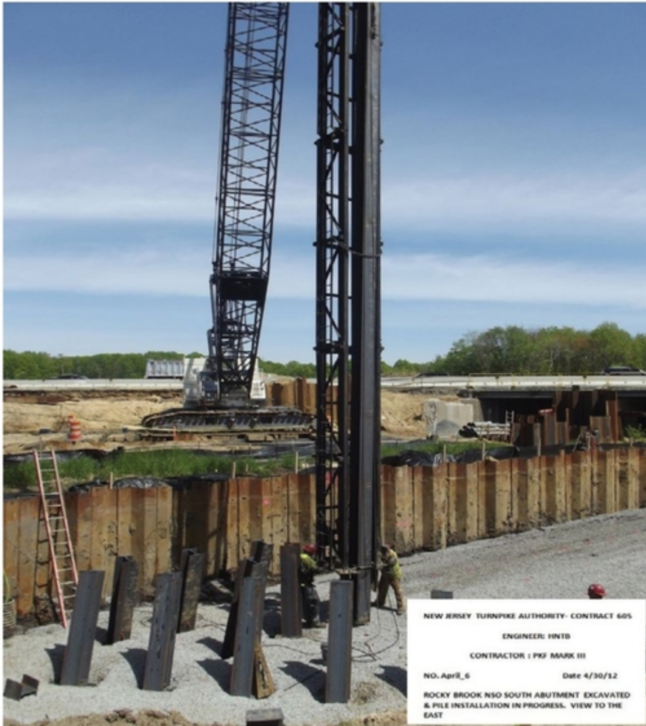
Figure 1: PKF piling crew driving production piles, Contract 605
