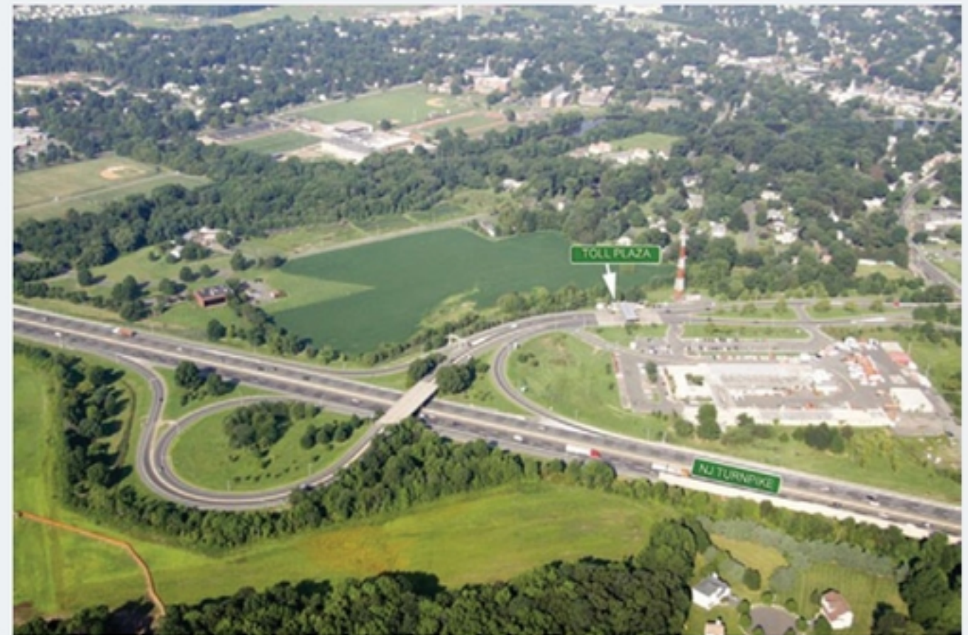
Section 6 – Preconstruction photograph of Interchange 8 located west of the New Jersey Turnpike in East Windsor. A new Interchange 8 will be built on the east side of the New Jersey Turnpike during the Interchange 6 to 9 Widening Program.
