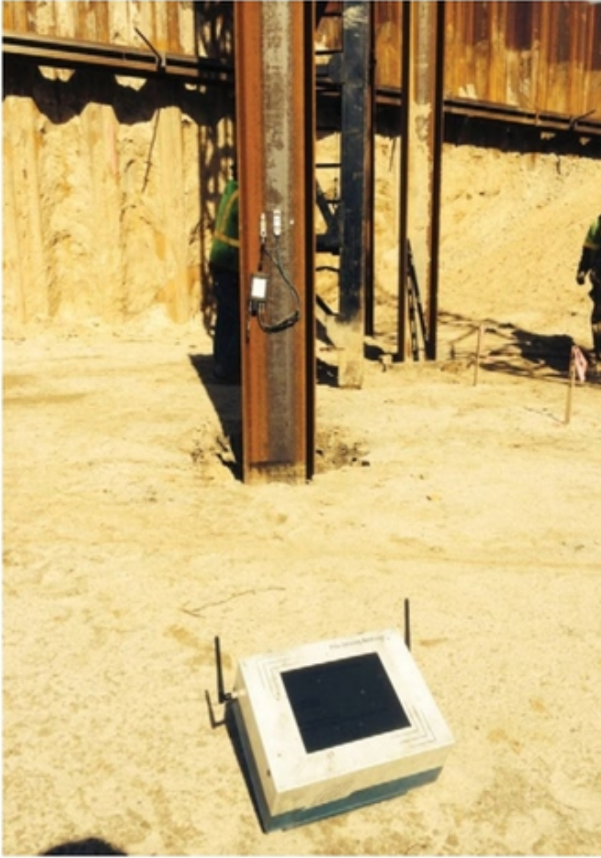
Figure 3: Pile Driving Analyzer® during restrike testing
