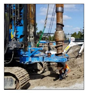
Figure 1. DDP drilling rig used on the project.
