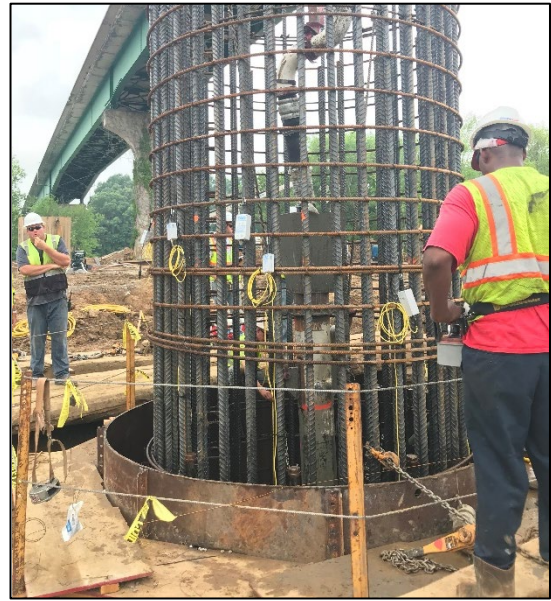
Figure 12. TAG and TAP Edge units on wires.
