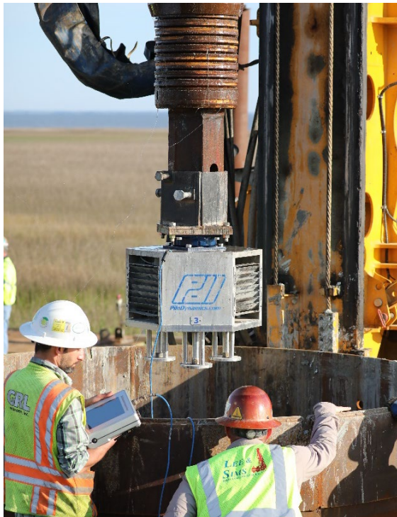
Figure 32. SQUID moving over shaft excavation.
