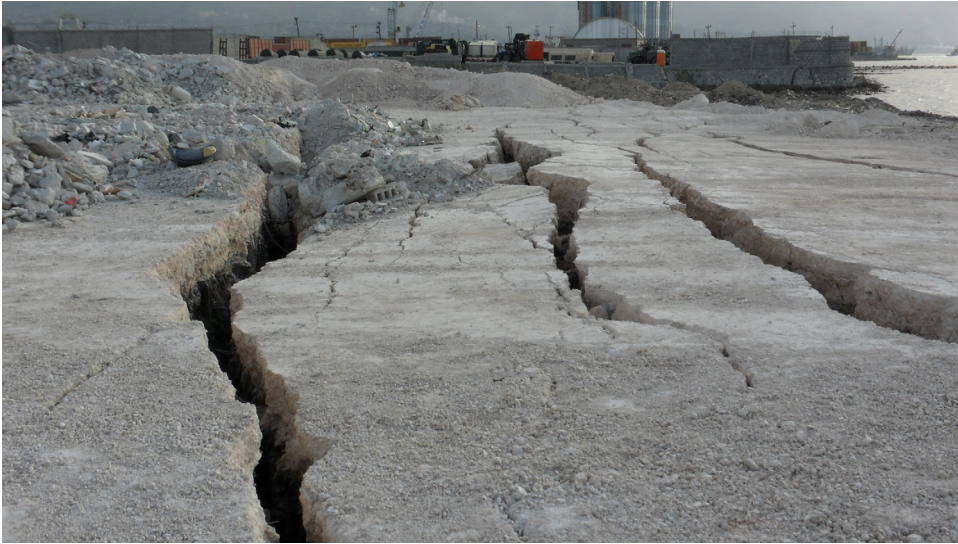
Figure 11. Lateral spreading in the storage yards in the northern part of the port facility.
