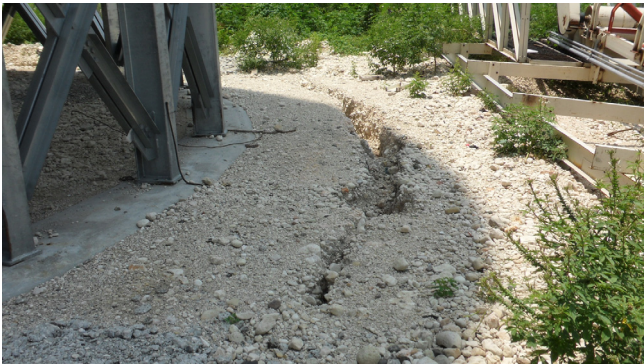
Figure 10. Crack in the soil around the base of the silos. This crack was likely made from uplift of the footing due to overturning moments induced by the earthquake shaking.
