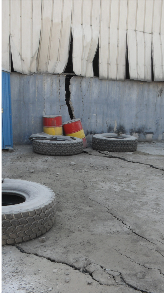
Figure 7. Lateral spreading crack extending into the western foundation wall of the west warehouse.
