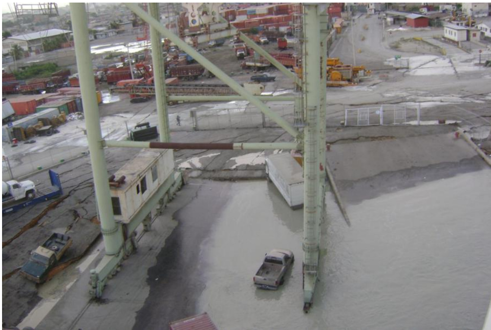
Figure 6. Photo taken immediately after the earthquake with the crane in its most eastward position and with the landside legs of the crane above water. Photo taken facing east. (gCaptain, 2010).
