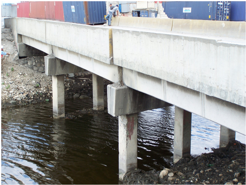
Figure 13. Minor crushing and lateral offset of middle and southern bridge spans for bridge connecting silo area to northernmost storage yards. Photograph taken looking northward.
