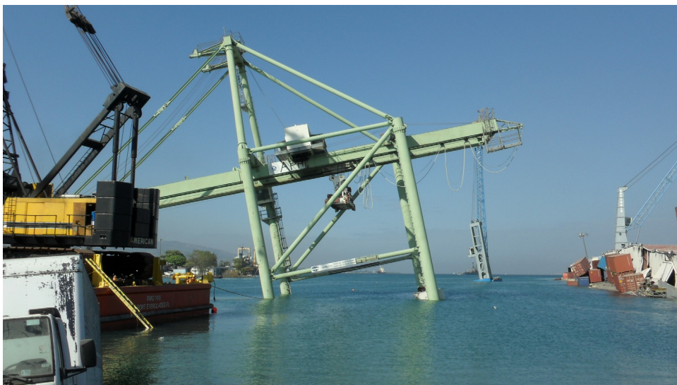
Figure 5. Submerged 15-m gauge container crane (foreground) and mobile crane (background).
