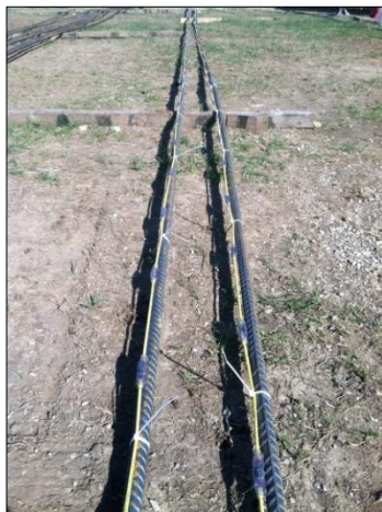
FIG. 12. Prepped Center Rebar
