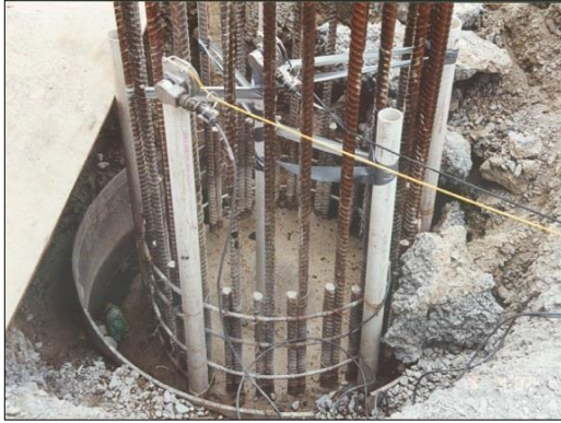
FIG. 3. CSL Tubes in Drilled Shaft
