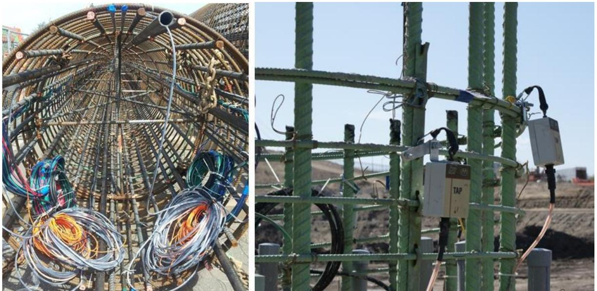
Figure 9: Thermal Wire cables installed in the cage (left), TAP data collector units connected in the cables (right)
