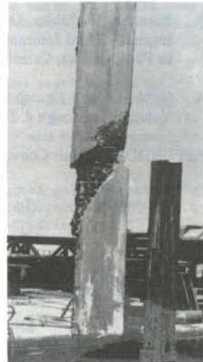
Figure 4: Pile Bottom Section after Extraction, Case 2
