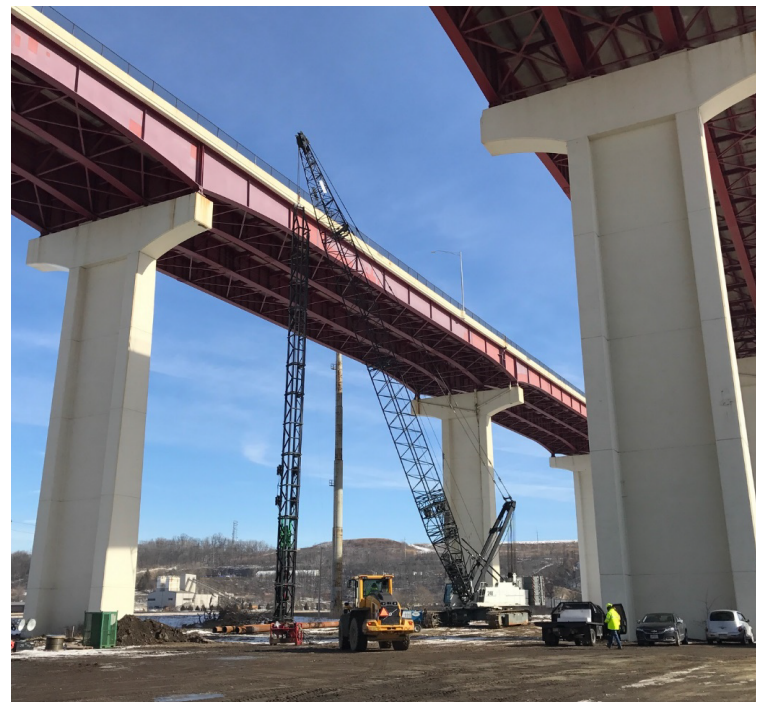
View of the I-480 Valley View bridge from job site
