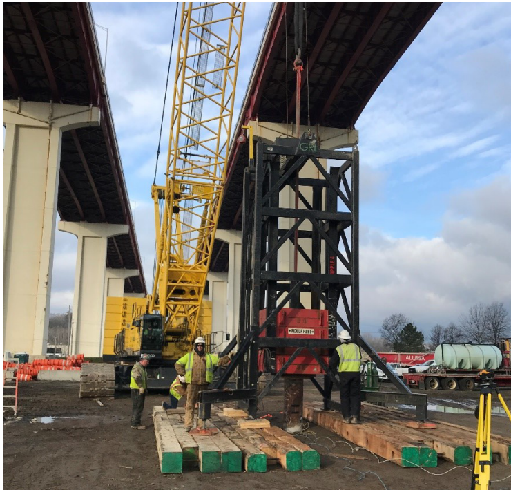
Preparing APPLE system for dynamic load testing on pipe piles
