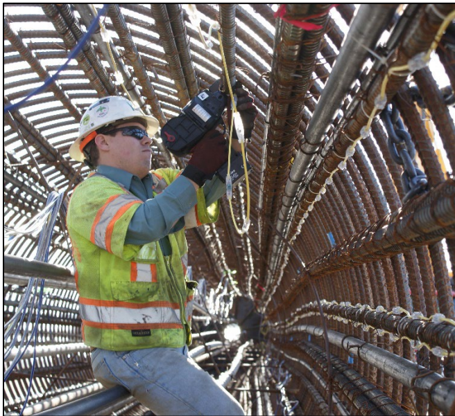
Figure 11. TIP wire attachment to reinforcing cage.
