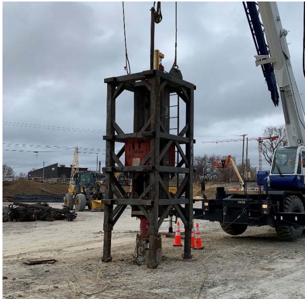
Figure 9. Drop weight system for drilled shaft testing
