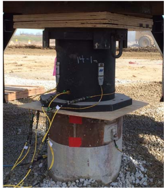
Figure 10. Instrumented drilled shaft for HSDPT
