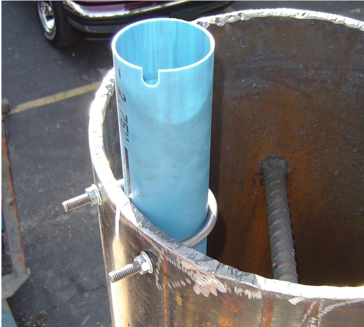
Figure 2. Inclinometer Casing Installed in Closed-End Pipe Pile Prior to Concreting.
