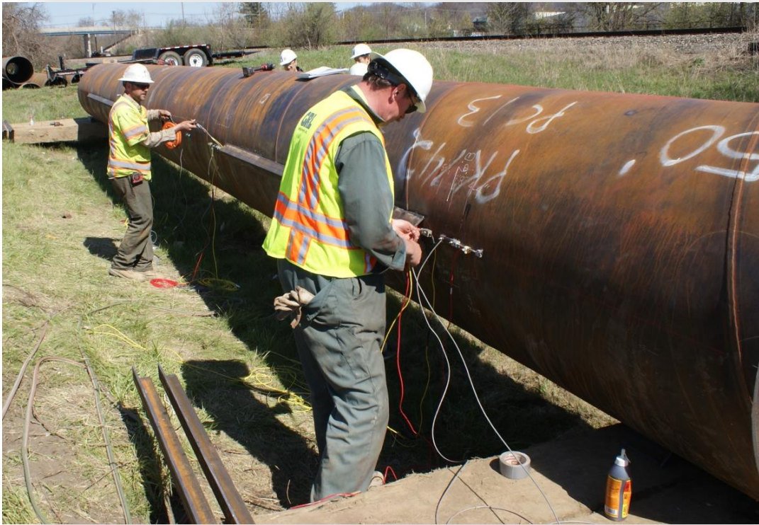
Figure 5. Attaching Instrumentation, Wiring, and Protective Cover Plate on Open End Pipe Pile.
