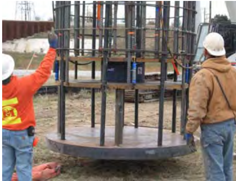
Fig. 5. O-cell and tube-a-manchette system in rebar cage
