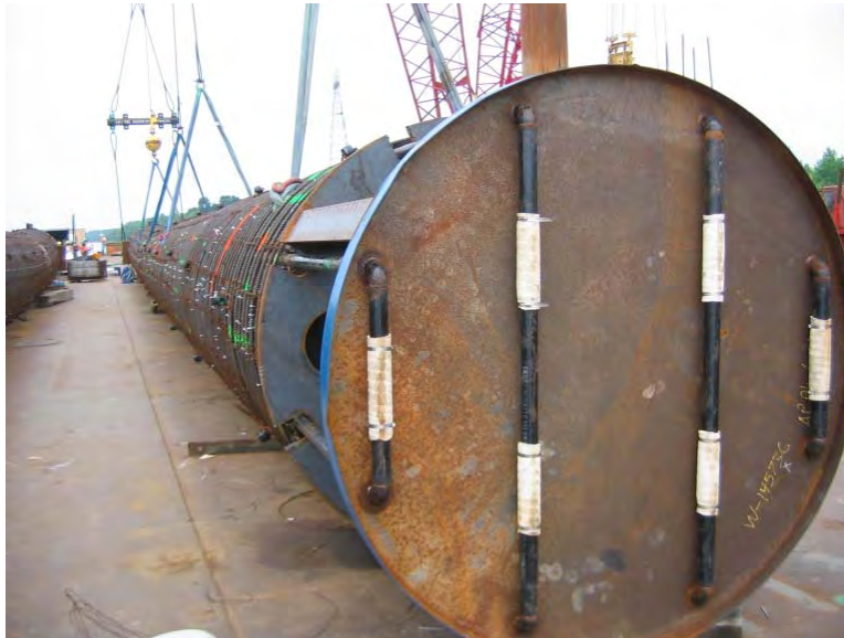
Fig. 2. Typical base grouting apparatus installed at the cage tip.
