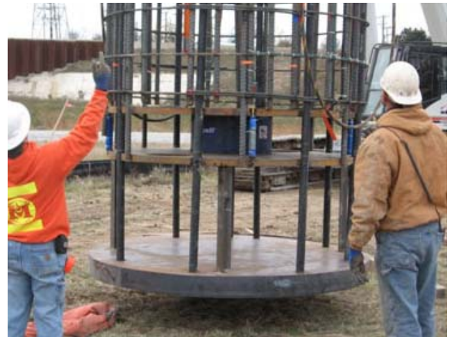
Fig. 7. O-cell and tube-a-manchette system in rebar cage
