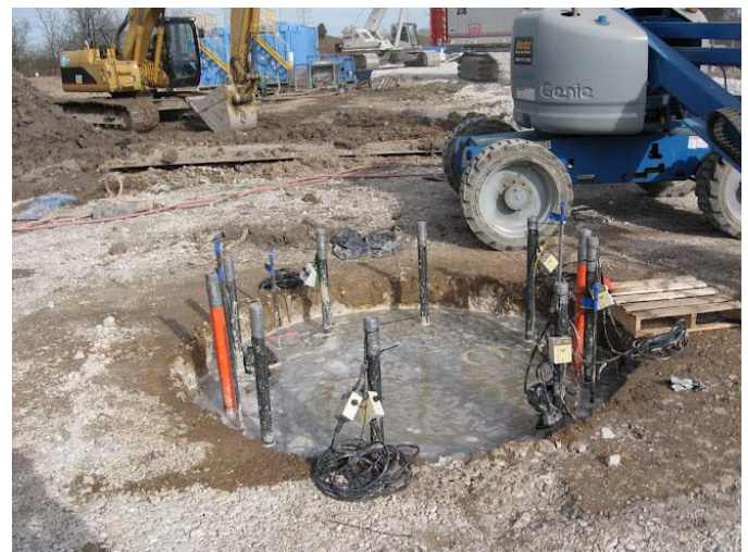
Fig. 8. Installed Test Shaft CTS-1
