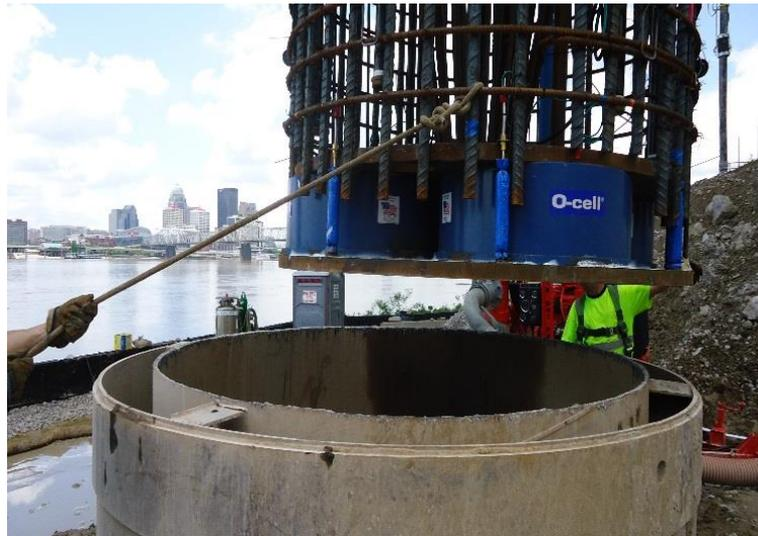
**Figure 6 O-cell assembly at the tip of reinforcement cage being installed into the test pile excavation**
