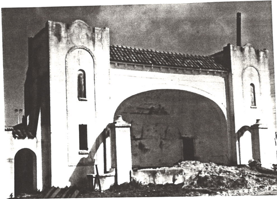
Figure 1: View of the building front
