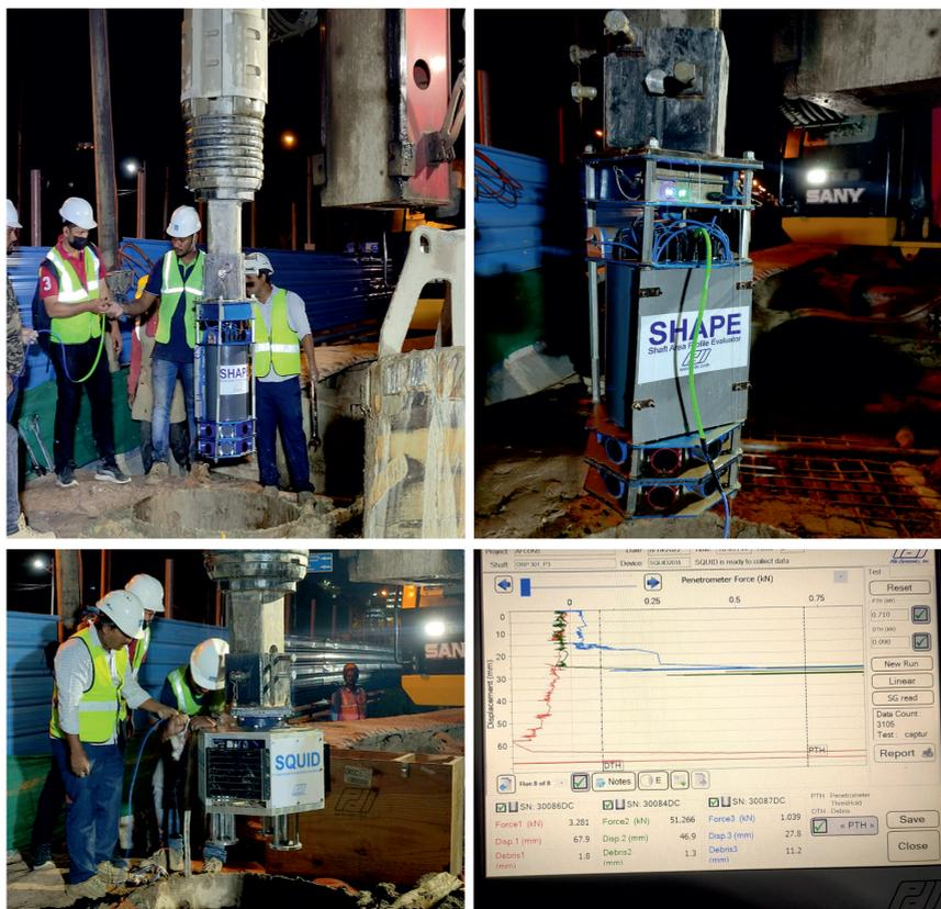
Figure 1: Site Photographs – Conduct of SHAPE and SQUID
