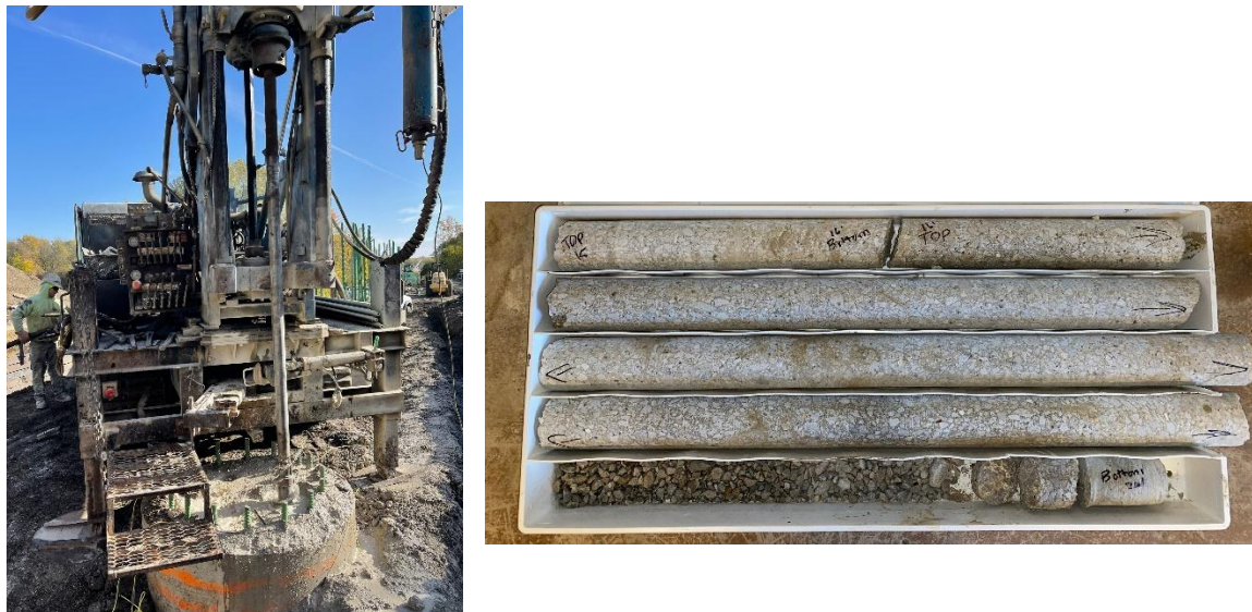
Fig. 9. Shaft 2 Coring Operation (left) and Retrieved Cores (right)
