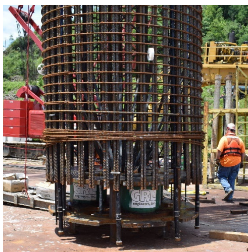
Figure 34. Multi-cell jack assembly in cage at base of drilled shaft.
