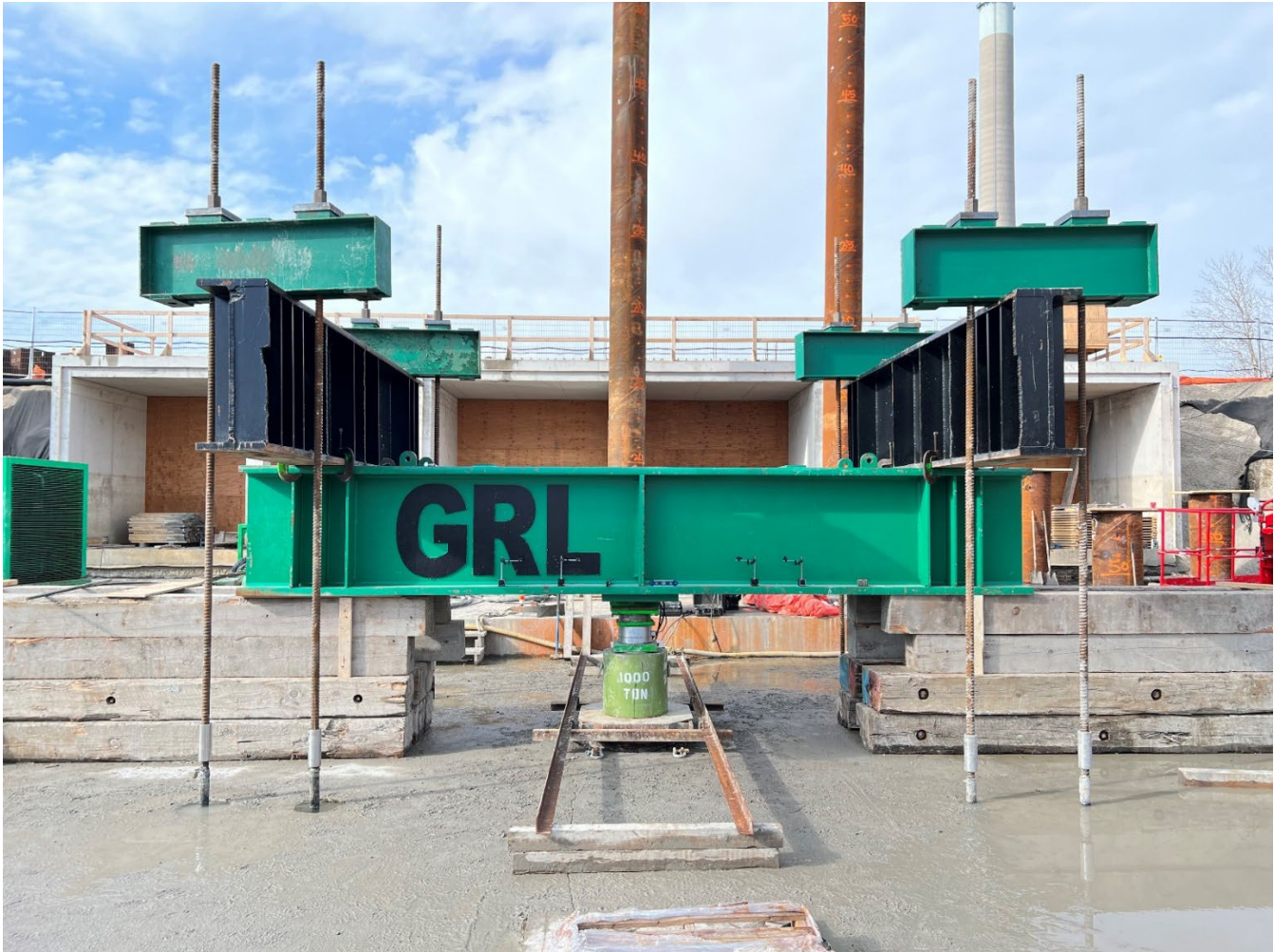
Figure 1. – Static Load Test 1000 ton reaction frame
