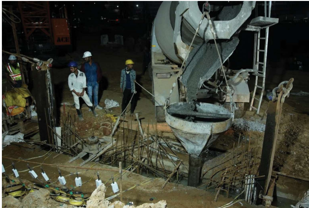
Fig.6 Concreting using Tremie method
