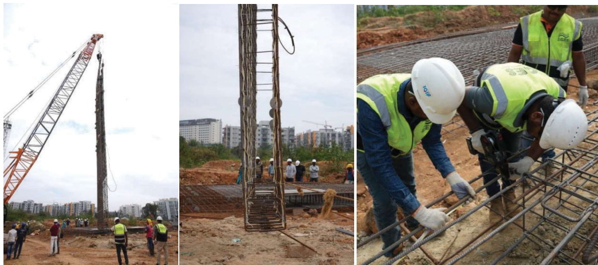
Fig.3 Thermal wires rigged up on panel-63
