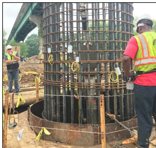
Figure 14. TAG and TAP Edge units on wires.
