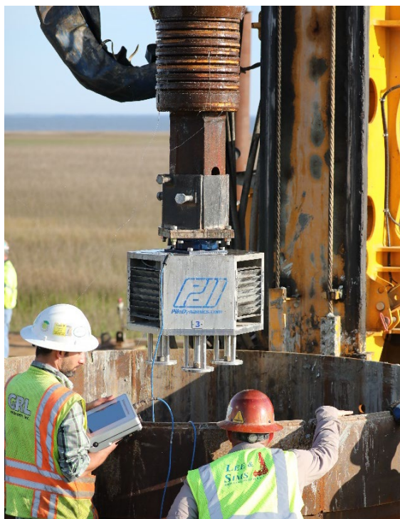
Figure 43. SQUID moving over shaft excavation.
