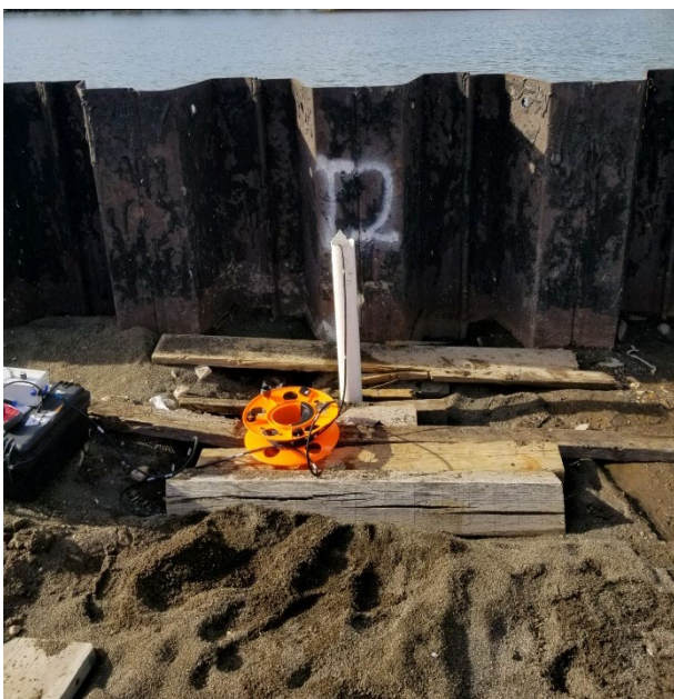
Figure 54. LITE probe in PVC borehole.
