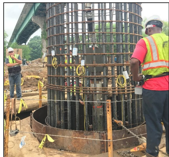
Figure 14. TAG and TAP Edge units on wires.
