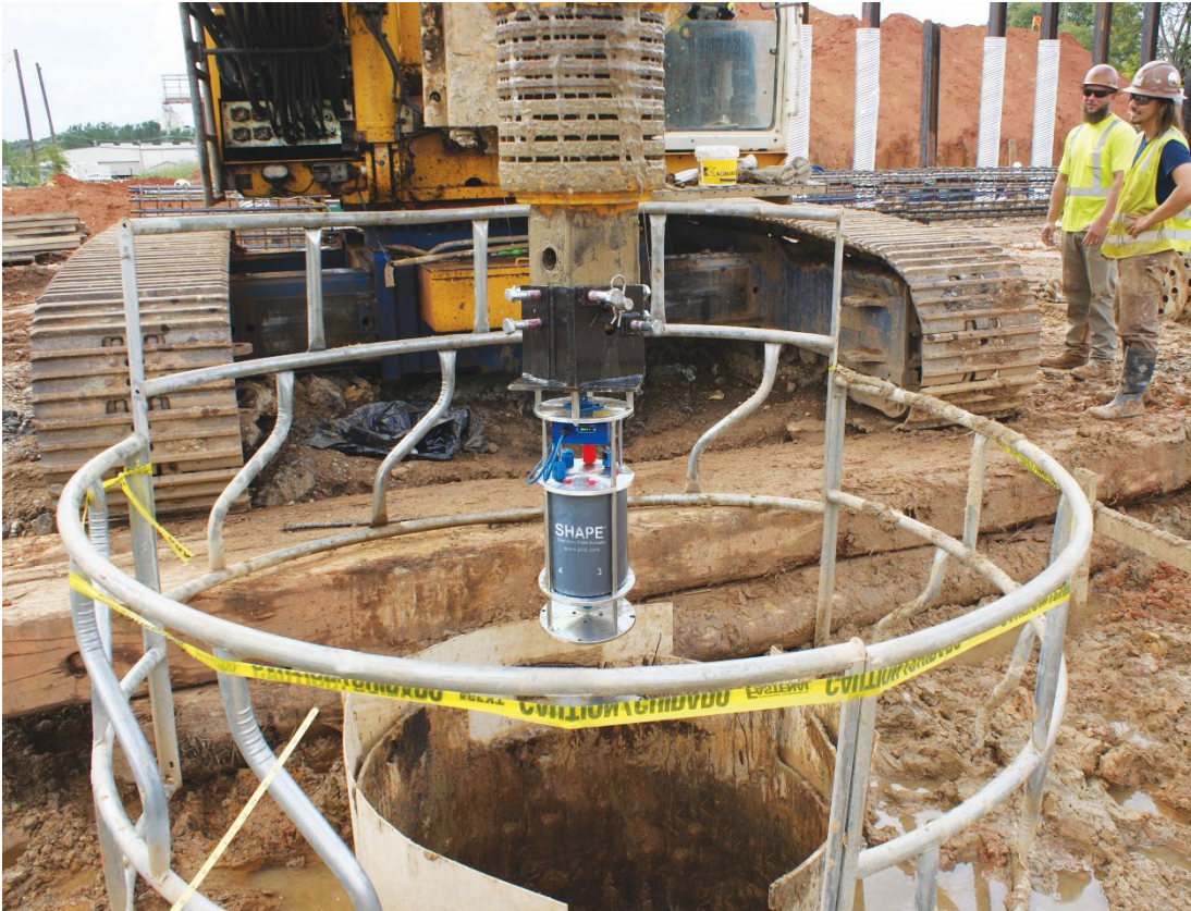
Figure 40. SHAPE moving over shaft excavation.
