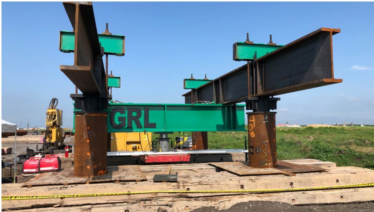
Figure 27. Reaction pile load frame for an axial compression load test.
