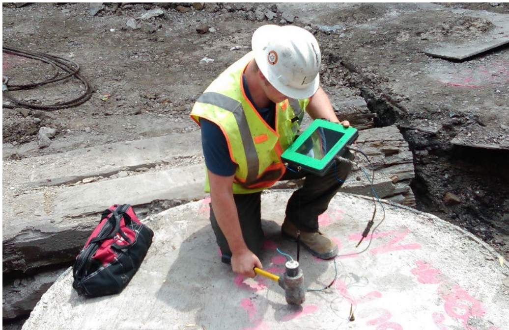
Figure 25. Low strain pile integrity test
